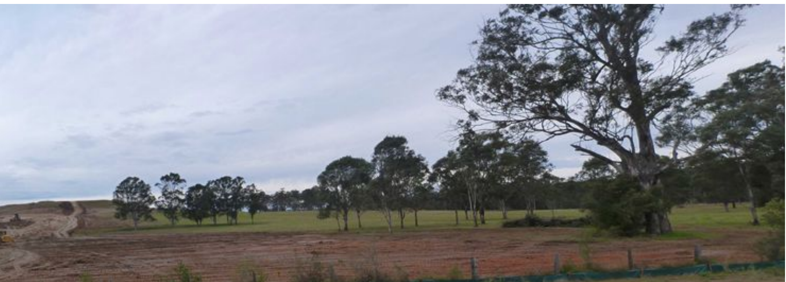
Broad-scale clearing for the Growth Centre precinct at Oran Park. Photo Supplied.
